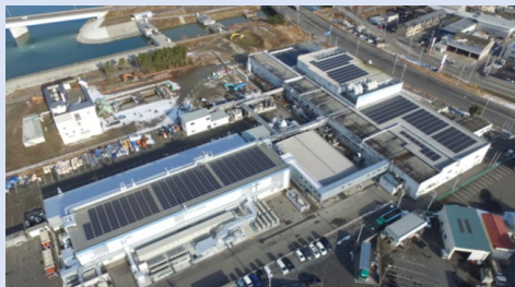
Ishinomaki Factory Commenced operation in March 2023 400kW 200t/year-CO2 reduction
