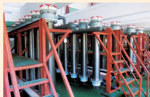
Photo: Soft etching waste liquid processing equipment in Guangzhou Plant.
