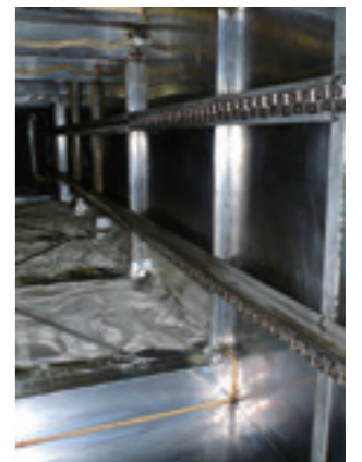
The drying oven interiors covered with rust and dust were also thoroughly cleaned.
