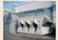
New air conditioning
