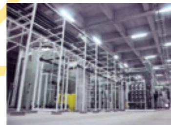
Reverse osmosis water refining equipment
