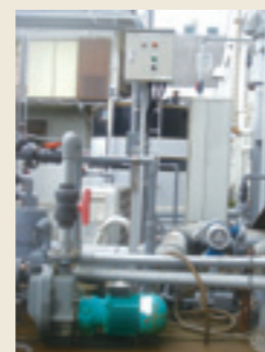
Waste acid liquid treatment device
