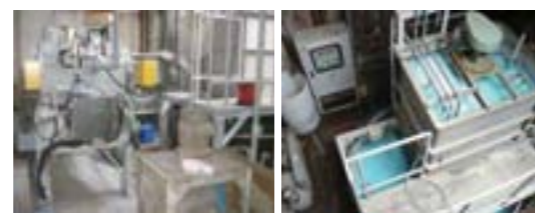
Waste alkali liquid treatment device at the Kanagawa Plant
