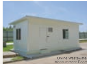
Online Wastewater Measurement Room
