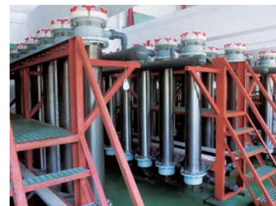
Photo: Soft etching waste liquid processing equipment in Guangzhou Plant.
