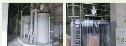
Reactor tanks (reacting process) Centrifuge
