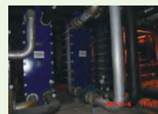
Photo: Heat exchanger
